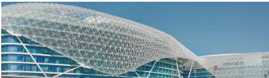
YAS MALL - SKYLIGHT
